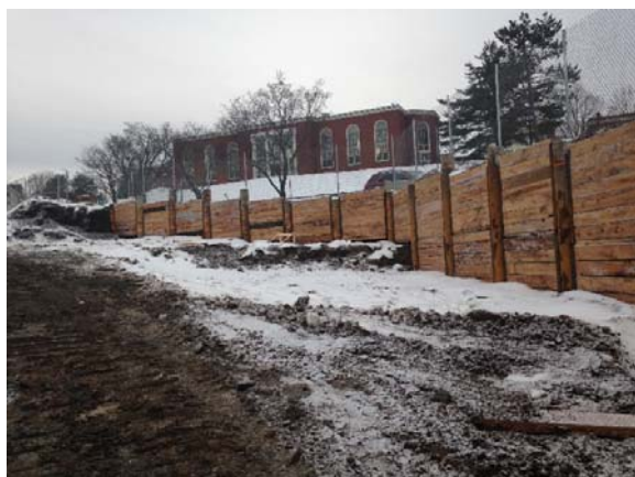
Installation of shoring along Mackay
