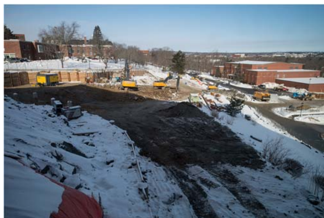
Mass excavation for building
