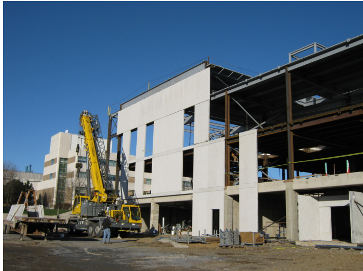
University Commons Construction Site, December 2010
