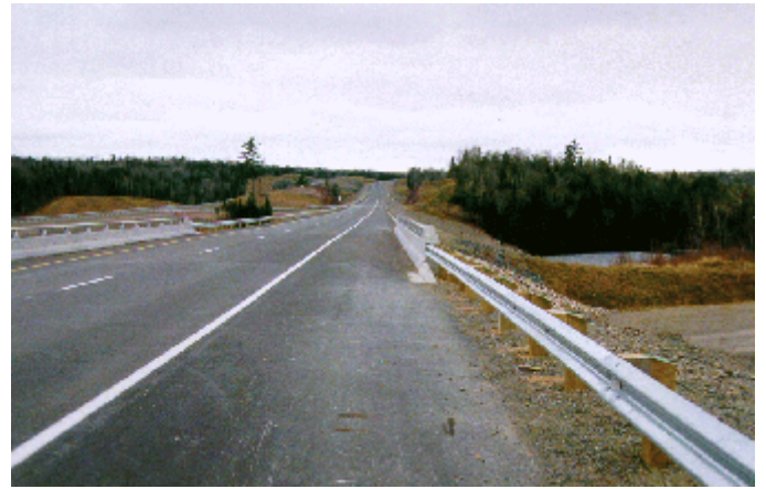
Photo 6: Shoulder width at Hillside Road
