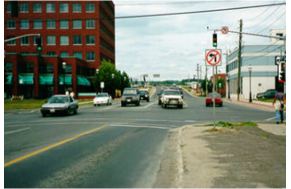
Photo 8. Misaligned intersection
