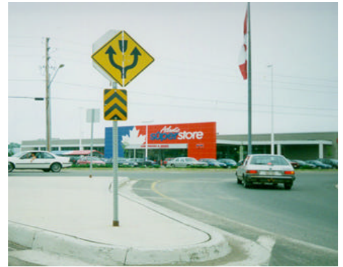
Photo 14. Communicates right-turn lane
