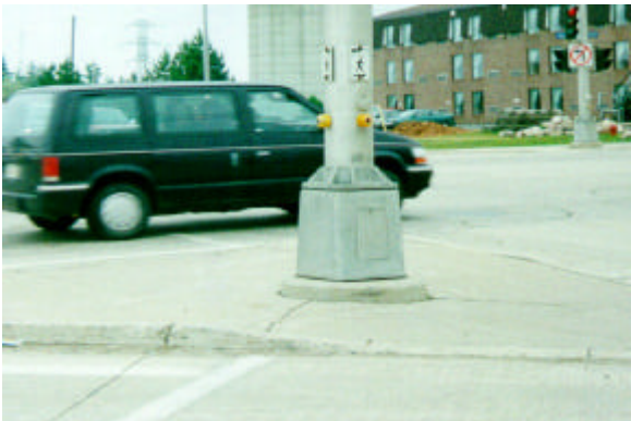
Photo 23. Raised breakaway support
