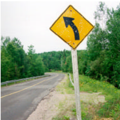
Photo 5. Cracked and non-retroreflective sign.
