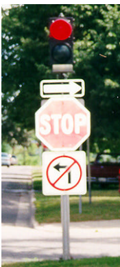
Photo 17. Faded Stop sign
