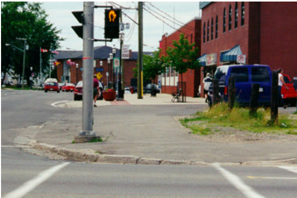
Photo 3. Inadequate curb cut-outs
