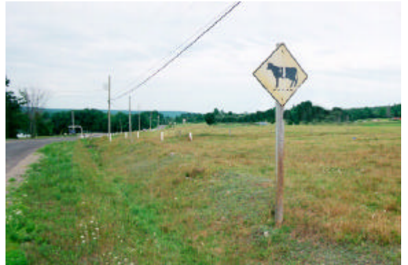
Photo 4. Cracked and faded sign; too much offset
