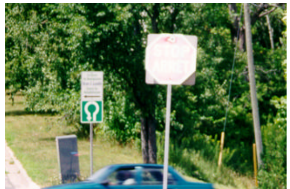
Photo 18. Faded Stop sign
