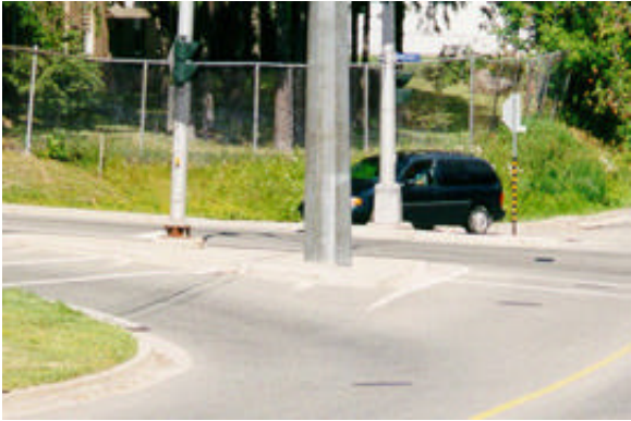
Photo 19. Exposed steel pole
