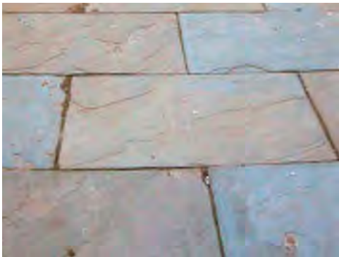
Limestone paving slabs were installed as part of a building renovation on the U.of T. campus.
