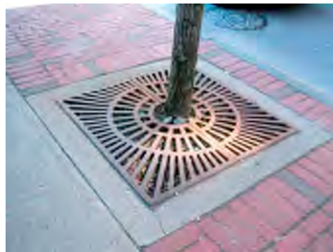
Metal tree grates in downtown Saint John prevent soil compaction while allowing water to penetrate roots.
