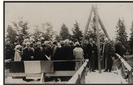
Laying the cornerstone of Memorial Hall, 1923. (UNB Archives and Special Collections, UAPC6no18)
