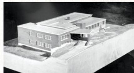
Both red and buff coloured bricks will be used in the construction of the building. The trim will be in cement or concrete. The roof will be flat but not all on one level. The entrances and the windows are particularly well designed.
