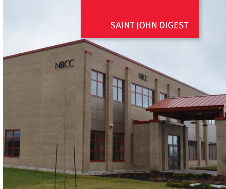
Above: NBCC building on the UNB Saint John campus. [Photo: Katie Bowden]
